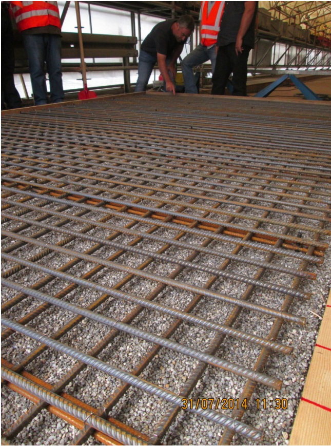
Reinforcing steel placed before HSC
