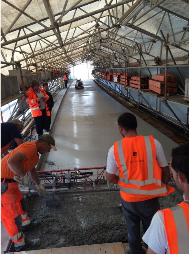
Pouring and smoothing HSC
