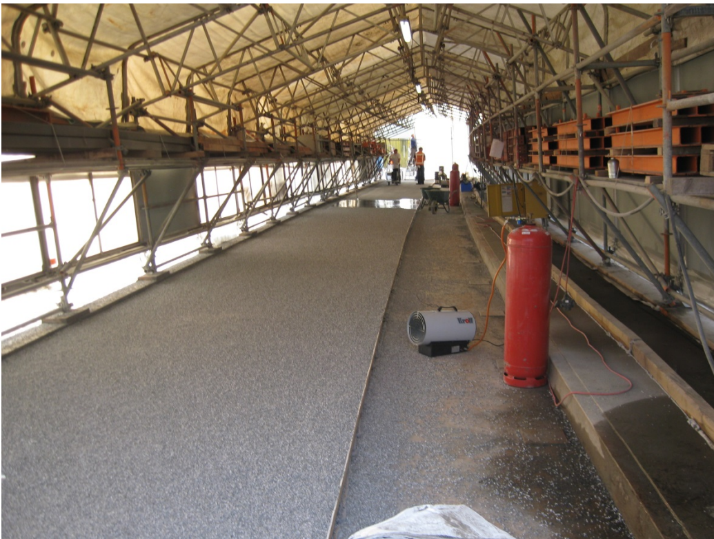
Surface treatment HSC with Epoxy Layer
